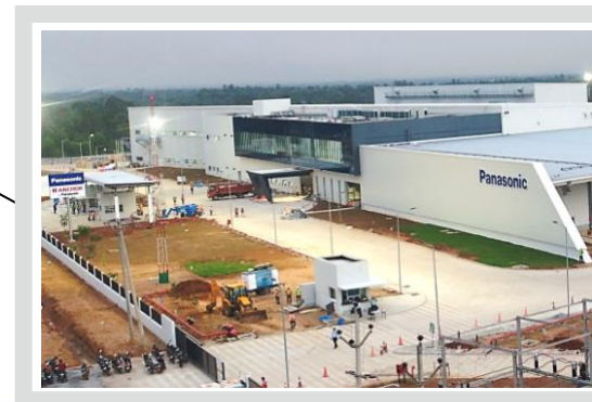
Sri City Factory Wiring Device
